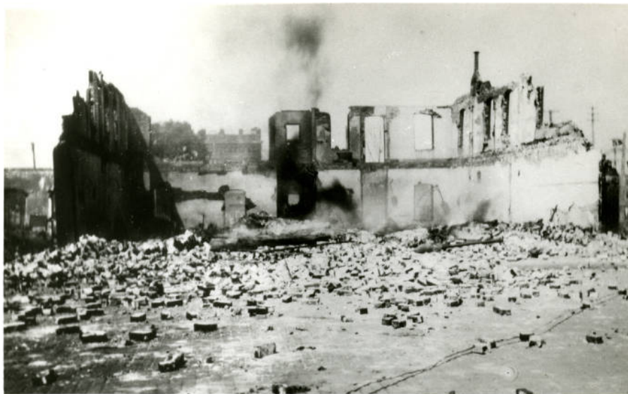
Figure 4. Remains of Dunbar Grade School following the 1921 attack on the Greenwood District. Photo courtesy of Oklahoma State University Library. https://dc.library.okstate.edu/digital/collection/TulsaRR/id/391/
